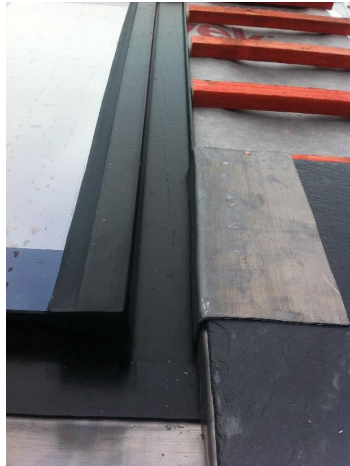
Lead soakers slate profile
